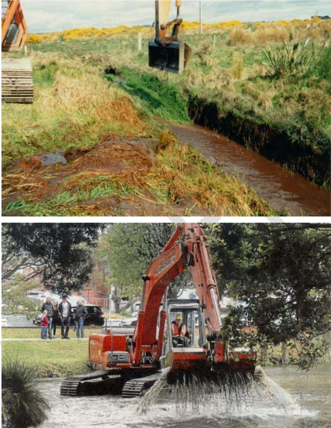
Figure 25 Hydraulic excavators are commonly used to remove sediment (and weeds) from the bank (Duck Creek) and inchannel (Avon River - Sunday Star Times 04 May 2014)
