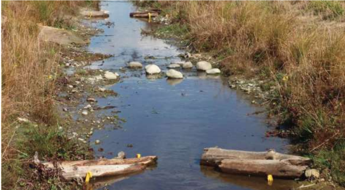
Figure 34 Addition of boulder clusters and logs for habitat diversity (CAREX Newsletter May 2015)
