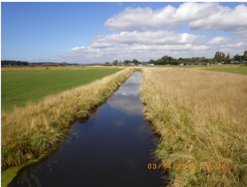
Taranaki Stream - Standing on the floodgate looking upstream
