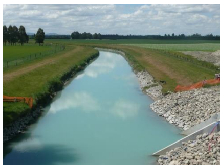
Photo: Environment Canterbury Water canal.
